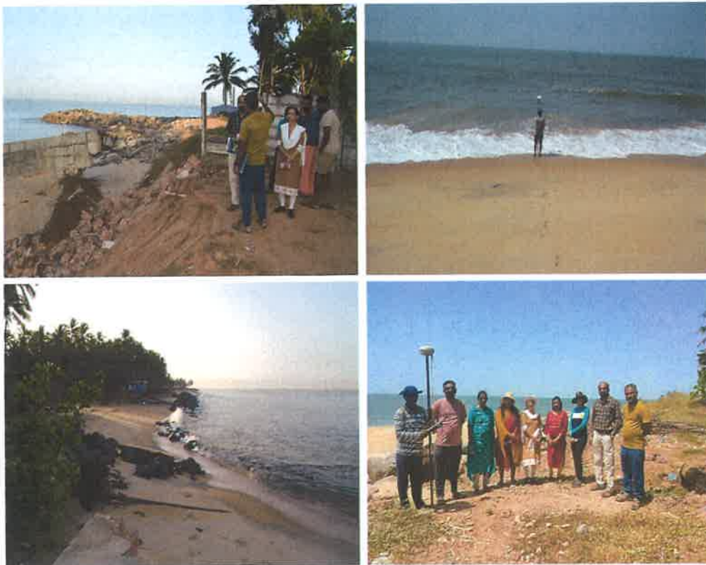
Figure 2: Field visit, discussions with officials, and field surveys were conducted along the Batapady coast in February 2024.
