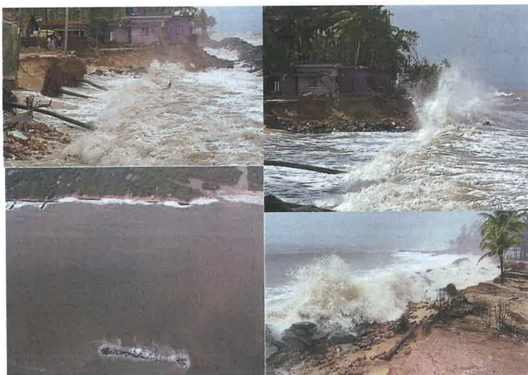
Figure 3: Field photographs of the wave action during the monsoon season and existing protection structures (offshore reef implemented previously) along the Batapady coast
